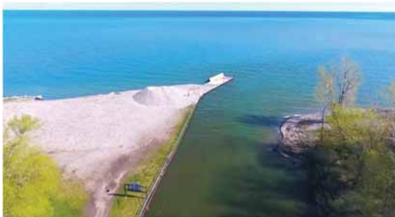
Pier, spoil area (dredged materials), and head of the east barrier bar
