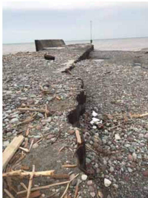
(b) Sediment deposit on and near the eastern edge of the pier
