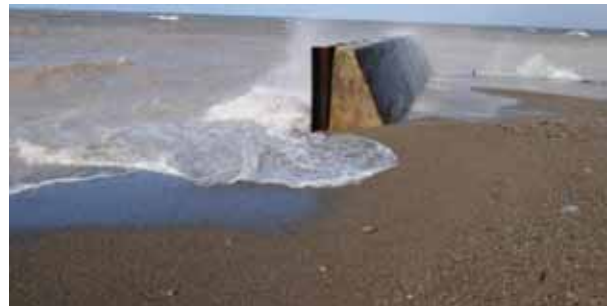
Looking north on the Pier during a winter storm; A portion of the materials that fill in the channel come over the top
