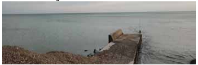
(a) Pile of gravel on the pier next to concrete wall from longshore sediment transport (LST); looking northeast
