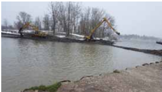
Dredging on Apr. 6, 2016; looking south
