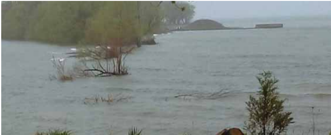
Breach widened in Apr. 2017 (~WL 247)
