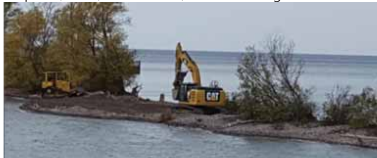
Repair completed in Nov. 2016 (~WL 244.4 IGLD85)
