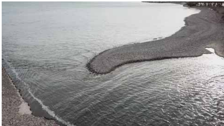
Looking east the pier/channel outlet before dredging, Mar. 27, 2018 (drone view) (~WL 245.5)
