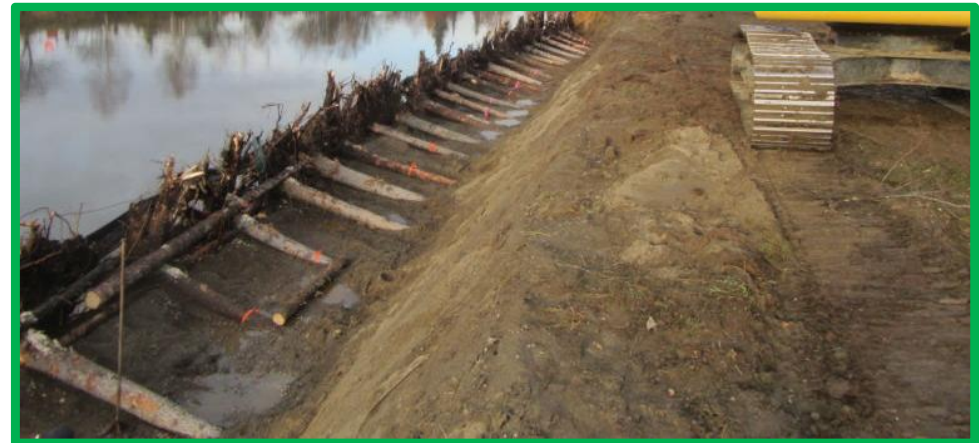
Installation of root wads; Imbedded into the revetment
